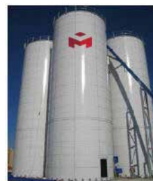
• Bulk Storage Silos
